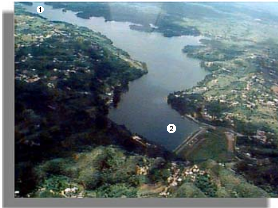
Figure 2-13. Location of sampling stations used in our monitoring program: 1) Entrance (USGS 50010720), 2) Dam (USGS 50010790).
